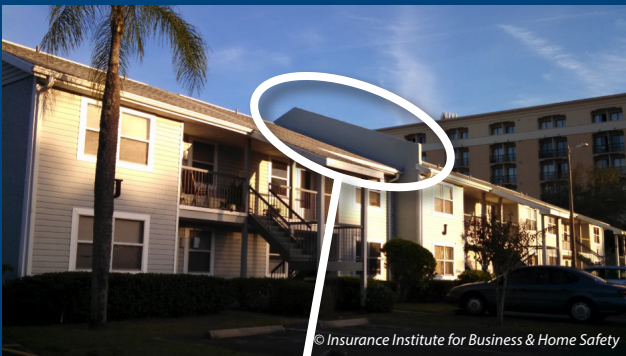
Fire wall separating two buildings – reducing the risk of a fire jumping from one roof to another
