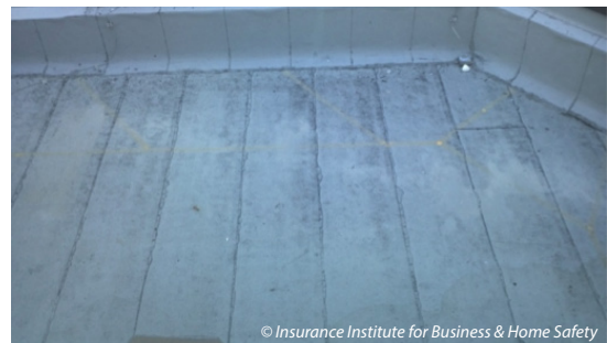
Modified bitumen roof cover.
